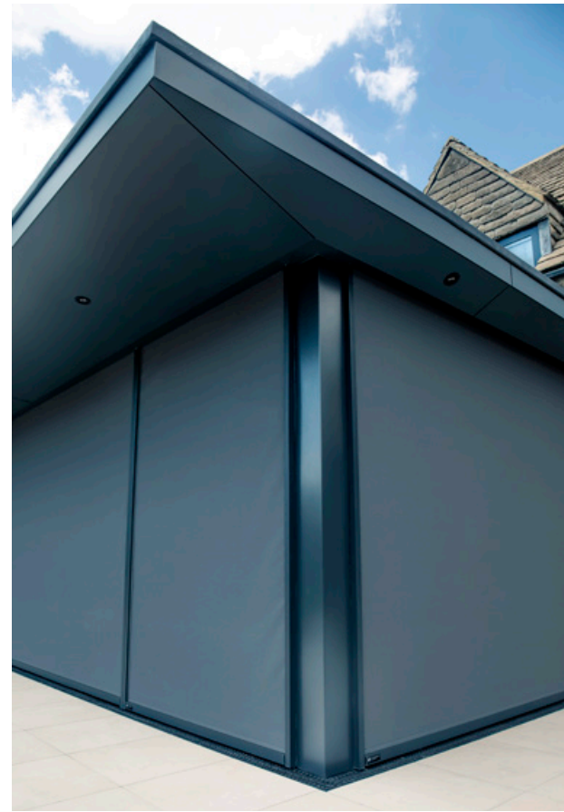
INTEGRATED WITHIN THE FAÇADE ↑
